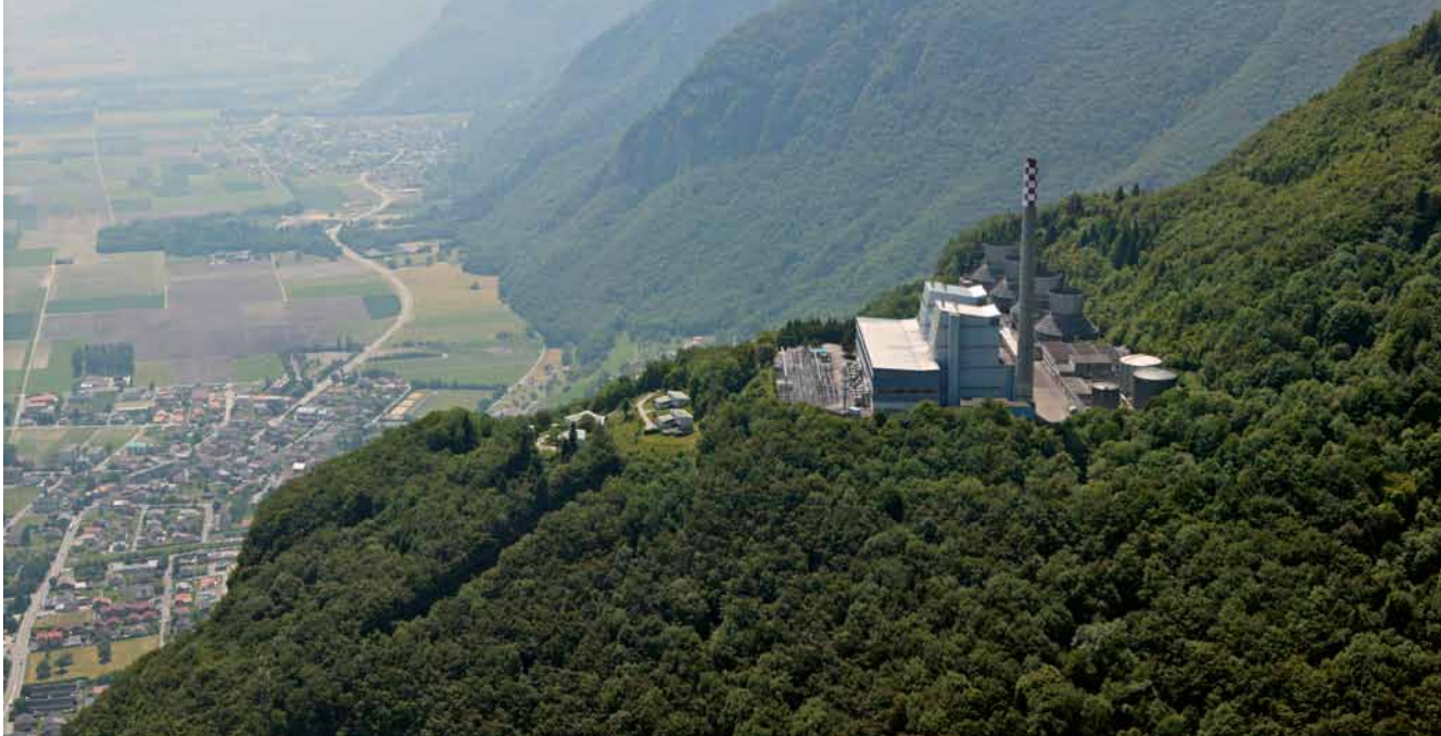
Centrale thermique de Chavalon Chavalon thermal power station
